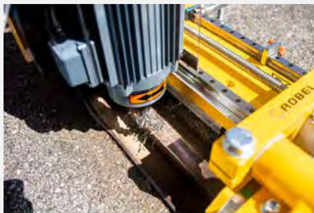
Drainage groove with ROFACE rail milling machine
