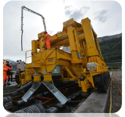
**Blend MXO8 mixer** was designed for the realization of the Monte Ceneri Tunnel: once finished (in 2020), this tunnel will reduce the travel time from Milan to Zurigo by about 1 hour and 15 minutes.
